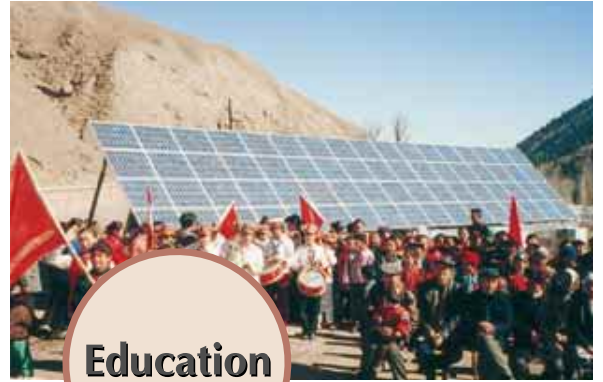
China : 4kW / School electrification (NEDO PROJECT)
